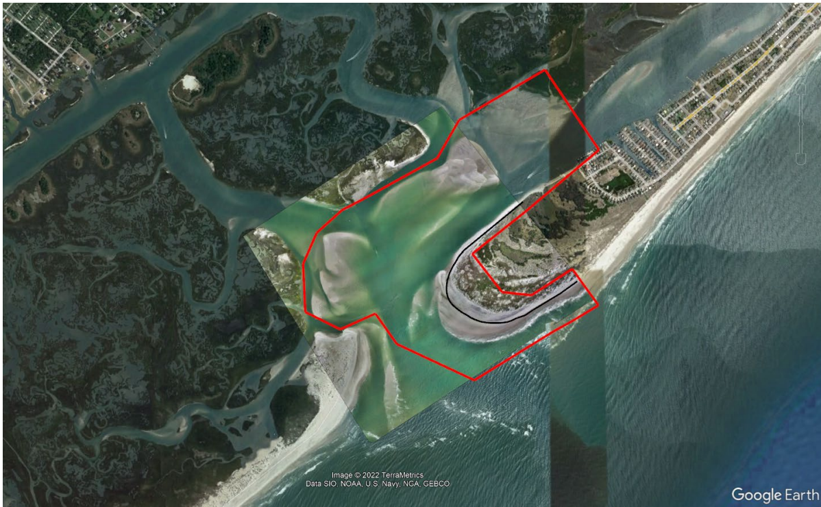
September 2022 Aerial Mosaic of Project Area (overlaid on Google Earth May 2021 Aerial)
